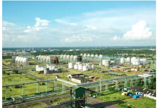
Hazardous chemicals storage in spheres & tanks
