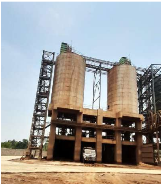
Fly ash storage silo
