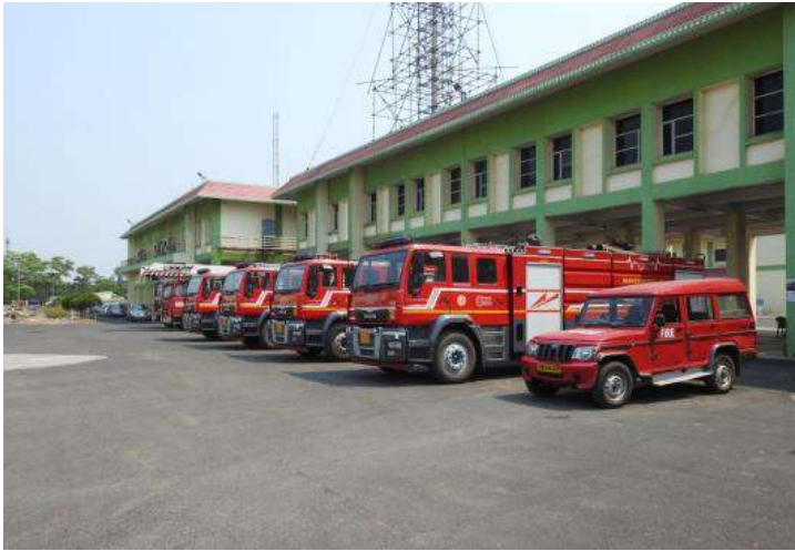
Fire fighting facility
